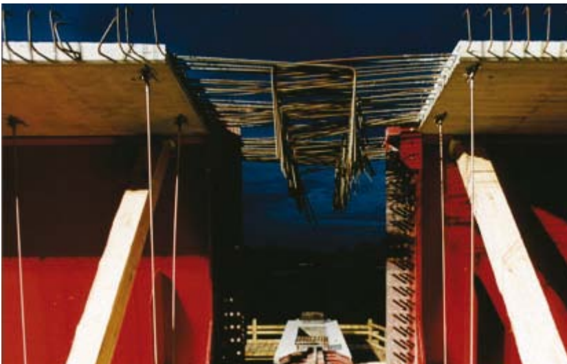
Fig. 11: Practical example: preparation for the concrete cross-beam over intermediate support – Oberhartmannsreuth Viaduct
