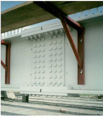
Fig. 24: Bolted strap joint of the main girder of a composite bridge in Istanbul, Turkey
