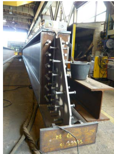
Fig. 13: Detail with a load distribution plate welded onto the bottom flange
