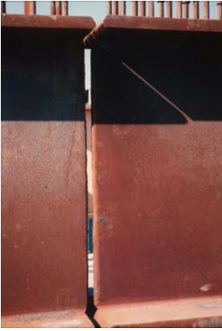
Fig. 21: Weld seam preparation for a welded butt joint of hot-rolled wide-flange beams for a composite bridge
