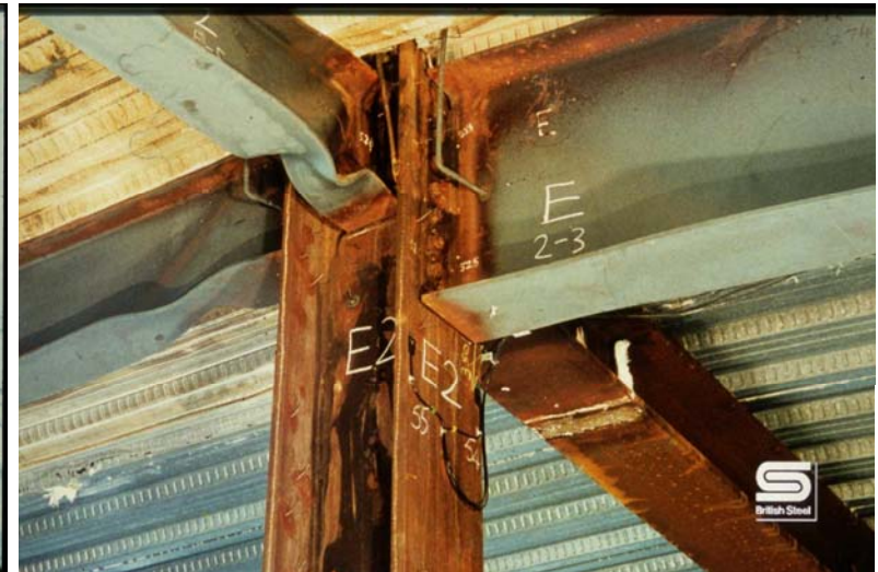
Deformed state of steel members around protected steel column
