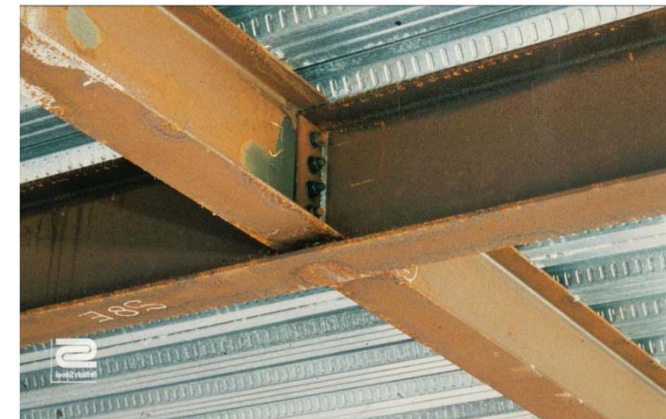
Beam to beam joint
