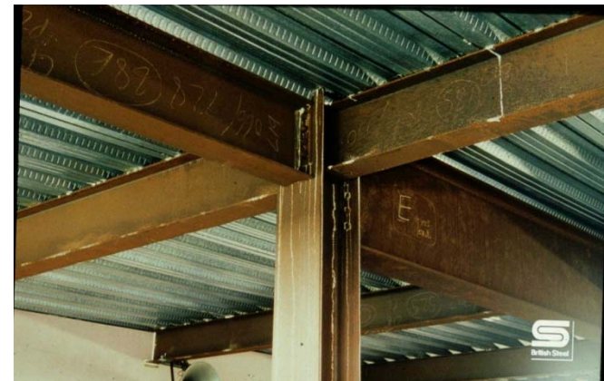
Beam to column joint
